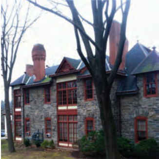
The Shields building, located behind the main residence, designed by Frank Heyling Furness and named for Mary Shields, an early benefactor of the Home for Consumptives.
